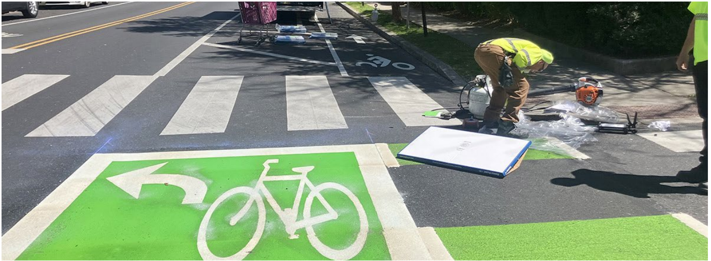
Workers add markings and a bike box on a separated bike lane in Lancaster. (Source: City of Lancaster )
